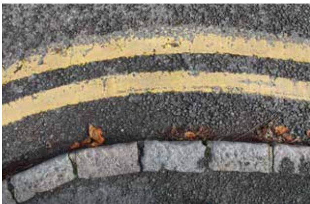
Figure 89: Stone kerbs along pavement
