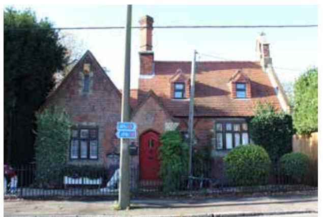
Figure 52: The Former School House
