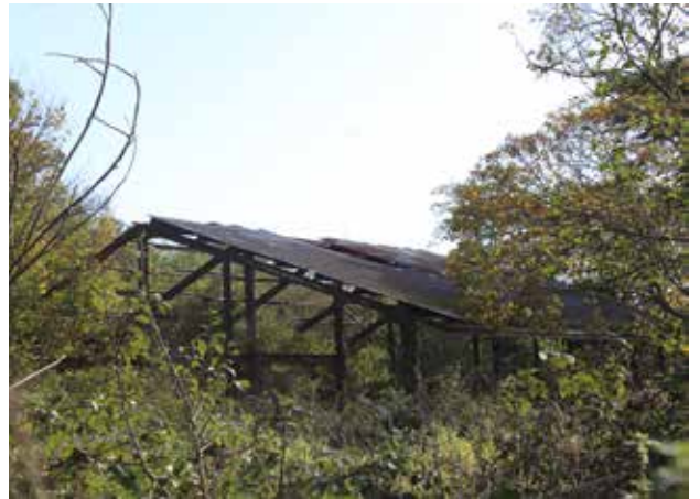
Figure 50: Structure remaining in the former Rectory grounds
